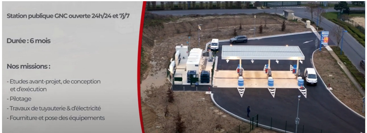
Figure 5 - Station GNC Vaux-Le-Pénil - source : TSG
